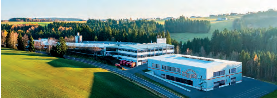
Wipro door and staircase factory in Vorderweißenbach
